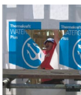
On arrival of doors and windows, cut Watergate at each opening on a 45° angle away from each corner. Pull the Watergate flaps inside and fasten to the inside of frame.
