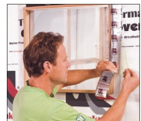
On arrival of doors and windows, cut the WATERGATE PLUS at each opening on a 45° angle away from each corner. Pull the WATERGATE PLUS flaps inside and fasten to inside of frame.
